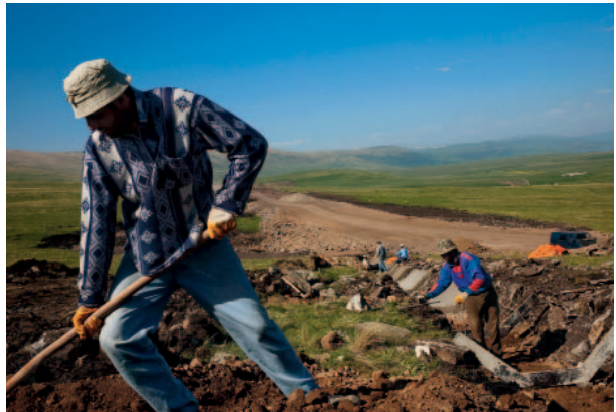
GEORGIA The railway provides work for many, including these men digging a drainage ditch along a freshly cleared railbed between Akhalkalaki and the Turkish border. Georgians (left) make the morning commute from the capital, Tbilisi, to jobs in nearby Rustavi in the existing railway's faded cars.
